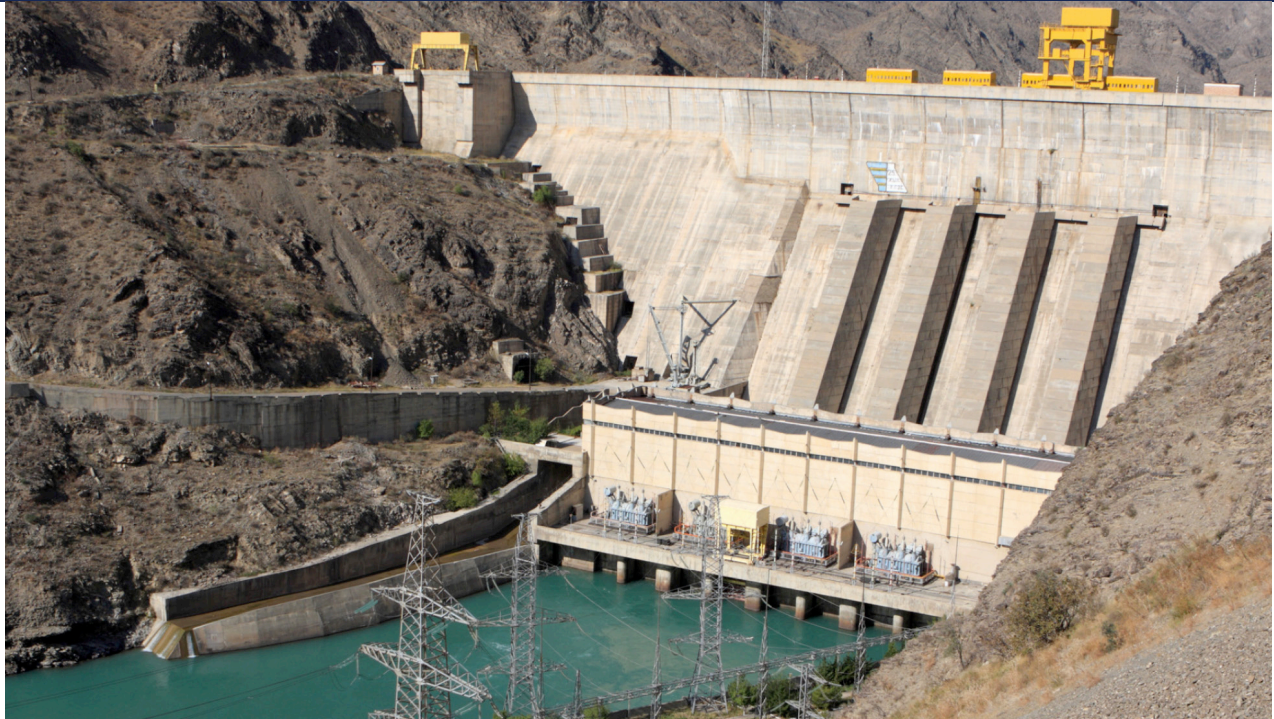
Figure 7 — Toktogul hydroelectric power station on Naryn River, Kyrgyzstan
