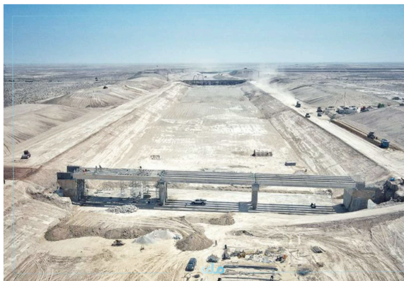
Figure 8 — Work in progress at the Qosh Teppe Canal
