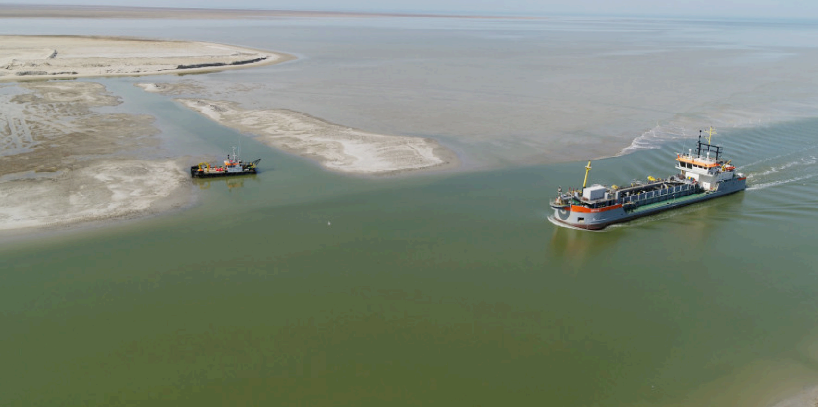
Figure 14 — Caspian maintenance dredging on the Prorva channel.
