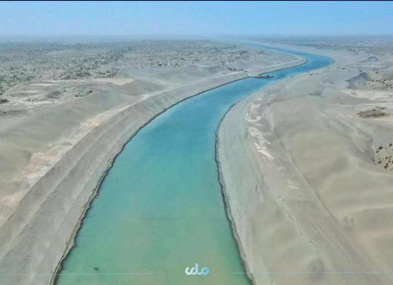
Figure 9 — Work in progress at the Qosh Teppe Canal
