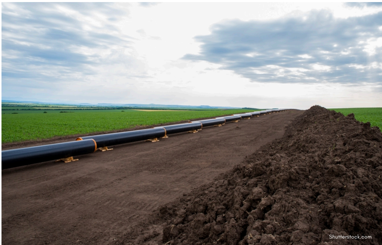
Work on the construction of the Greece-Bulgaria interconnector. Laying of natural gas transmission pipes
